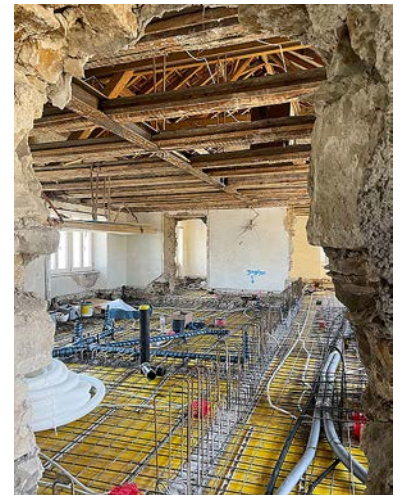
Neu-/Umbau MFH in Herznach
