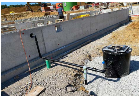
Neubau Stall in Wittnau
